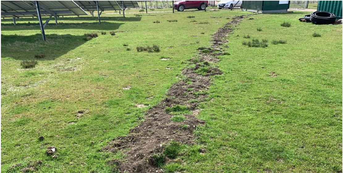
Insert 47: Trench During Wet Period
