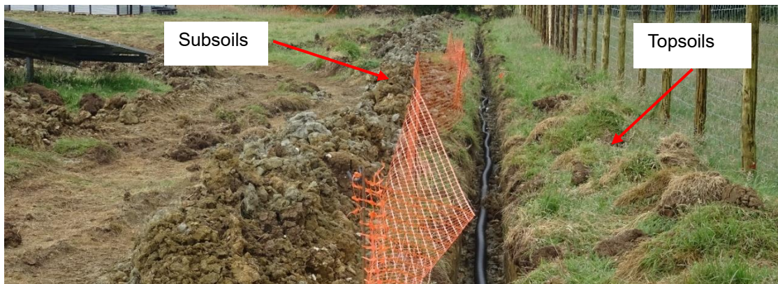
Insert 41: Subsoils Dug out of the Trench
