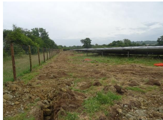
Insert 52: Topsoil Replaced
