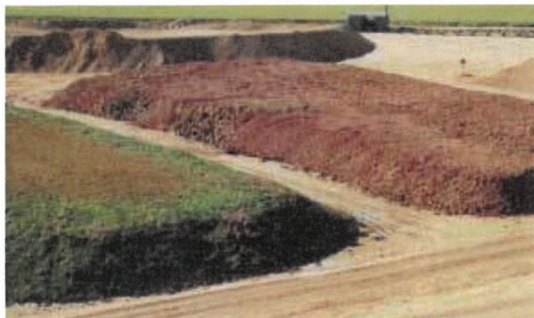
Clearly defined stockpiling of different soil materials
